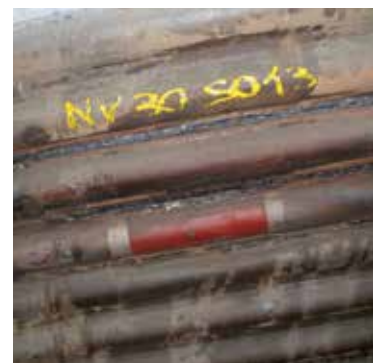
Built-in SMART Flux Sensor for measuring heat flow
